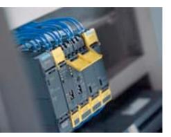
The new housing concept of the safety relays incorporates clearly labeled hinged covers, which facilitates sensor connection. In addition, you can add a seal to prevent parameters from accidentally being adjusted and to avoid time delays.
