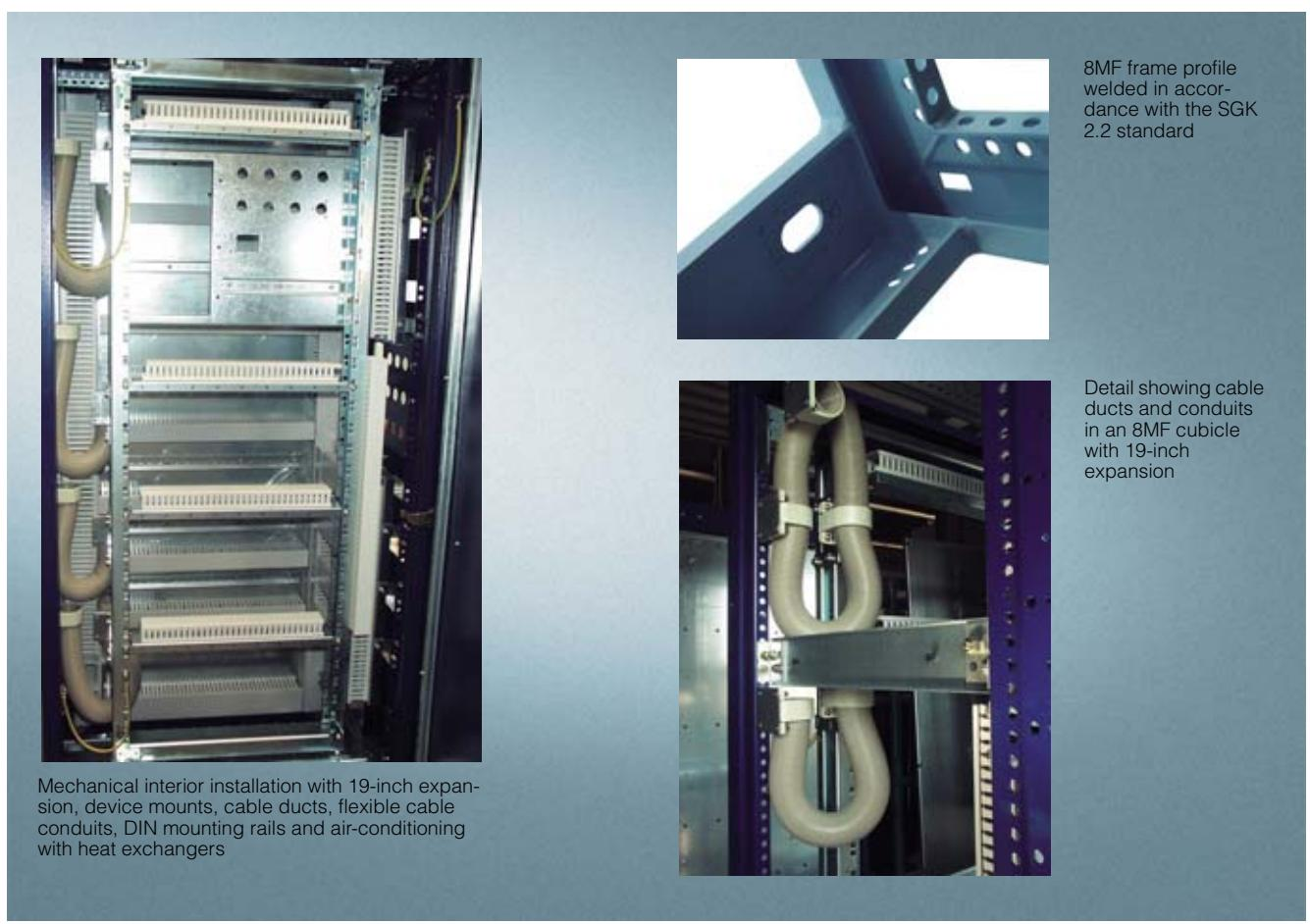
Mechanical interior installation with 19-inch expansion, device mounts, cable ducts, flexible cable conduits, DIN mounting rails and air-conditioning with heat exchangers
